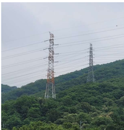
Figure 1. Towers on a mountain slope.
